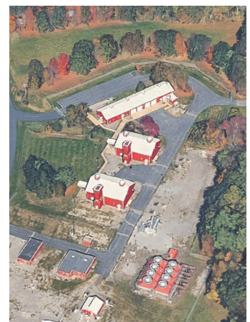
Wright Compressor Station - Source - Google Earth
